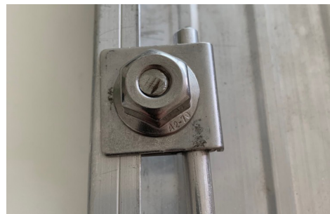
Anbindung Erdungsdraht an die Grundschiene Connection of ground wire to the base trough
