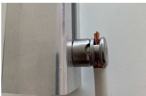
Anbindung Litzendraht an die C-Schiene Connection of stranded wire to the C-rail
