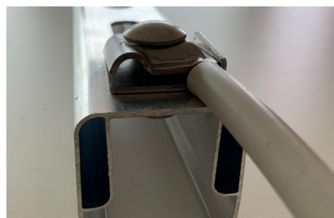
Anbindung Litzendraht an die C-Schiene Connection of stranded wire to the C-rail
